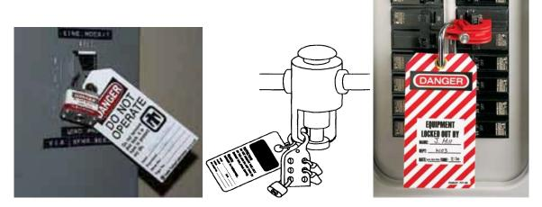
f. After ensuring that no personnel are exposed, and as a check on de-energized sources, operate the push button(s) or other normal operating controls to make certain the equipment will not operate. When working on electrical circuitry, test for de-energization with a meter.
